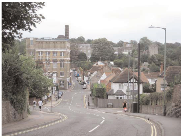
V1. Views east across the village from the higher ground to the west, including views along High Street and of the Church, Manor and former brewery
