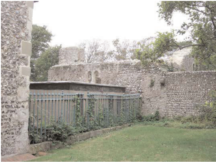
Fig 4 - View of old Manor from churchyard, with modern building
