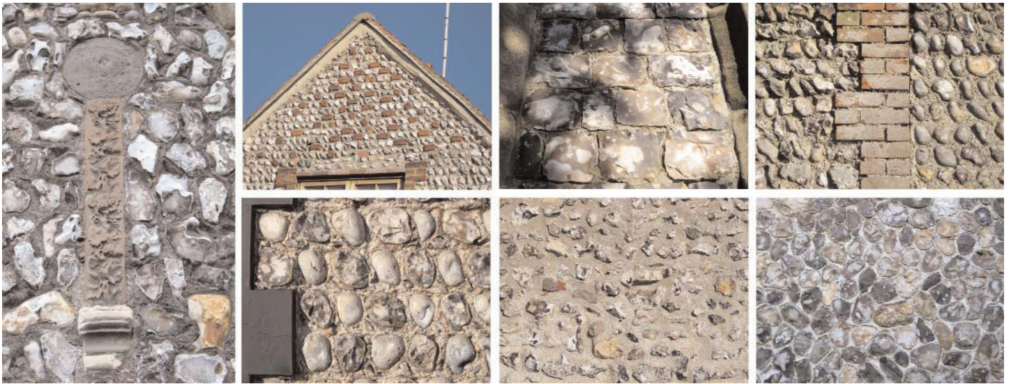
Fig. 17 - Types of flintwork in the Conservation Area
