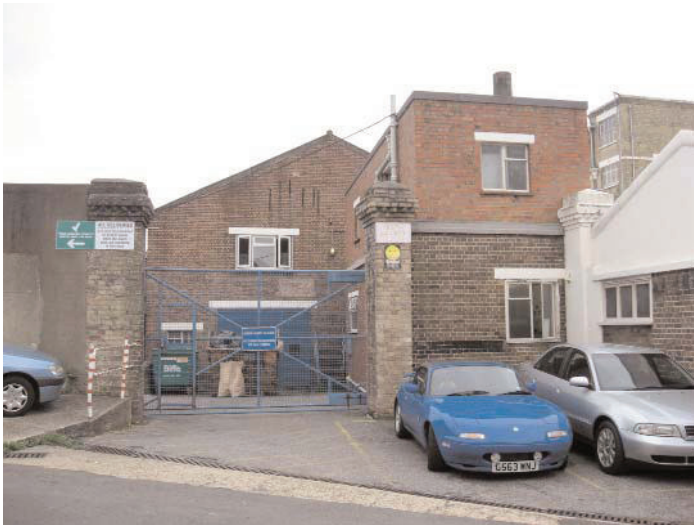
Fig. 13 - Tall boundary wall and accretions to rear of brewery
